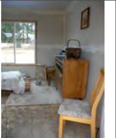
Photo 2.2: View of the northeast corner of burn cell 2
