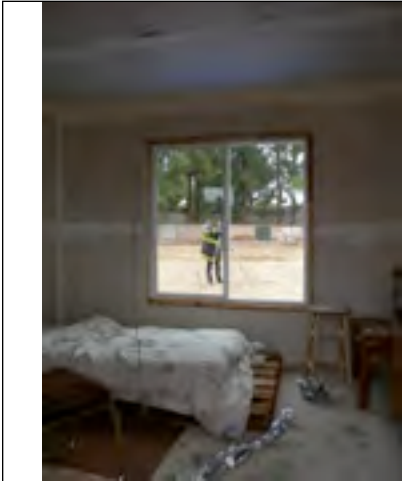
Photo 2.1: View of north wall of burn cell 2
