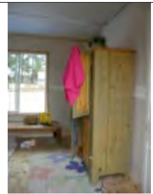
Photo 3.2: View of northwest corner of burn cell 3
