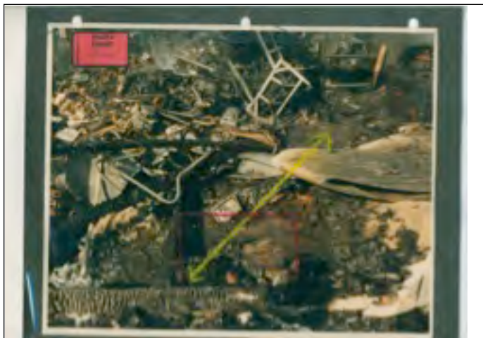
Photo 15: Low burning and hole in plywood subfloor at Graf fire (Exhibit 71)
