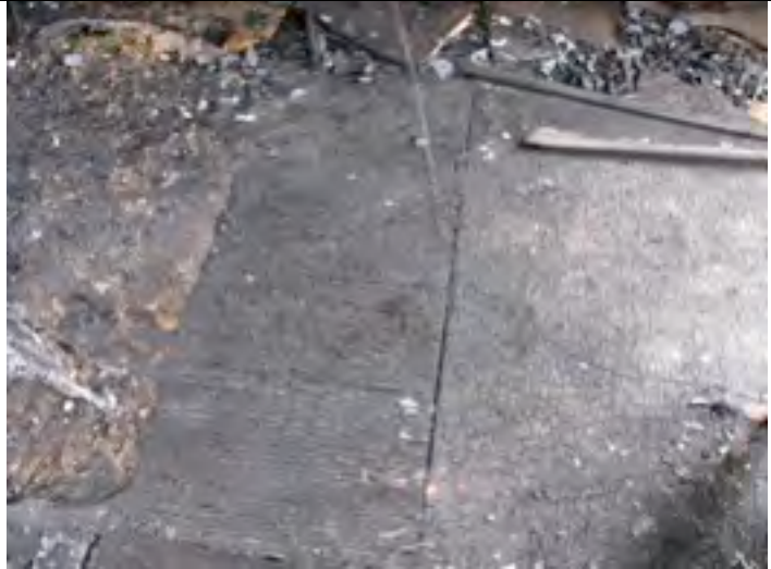
Photo 20: Floor burn patterns to plywood sheeting of burn cell #2.
