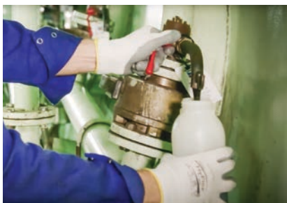
1. Collect drip oil samples from scavenge sampling valves.
